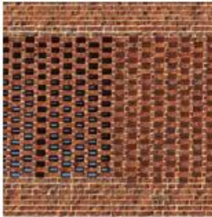
Perforated brick used for ventilation
