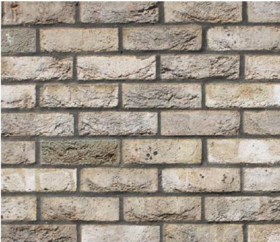
Buff brick with dark grey mortar used on the lower buildings
